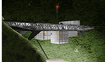
Prototype AMPZ-1045, Cultural Bridge for the City
